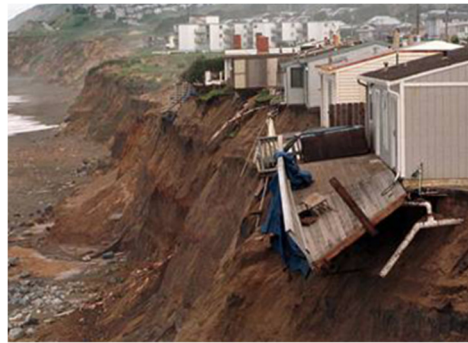
Homes built on a cliff near Pacifica, California collapse as ocean waves erode the cliff.
