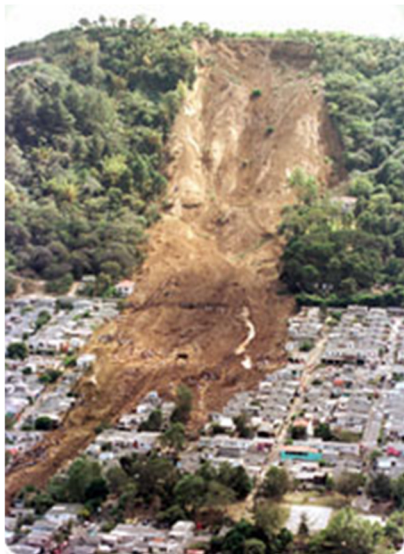
This landslide in El Salvador destroyed many homes in the valley below the hill. It happened after recent logging on the hill.
